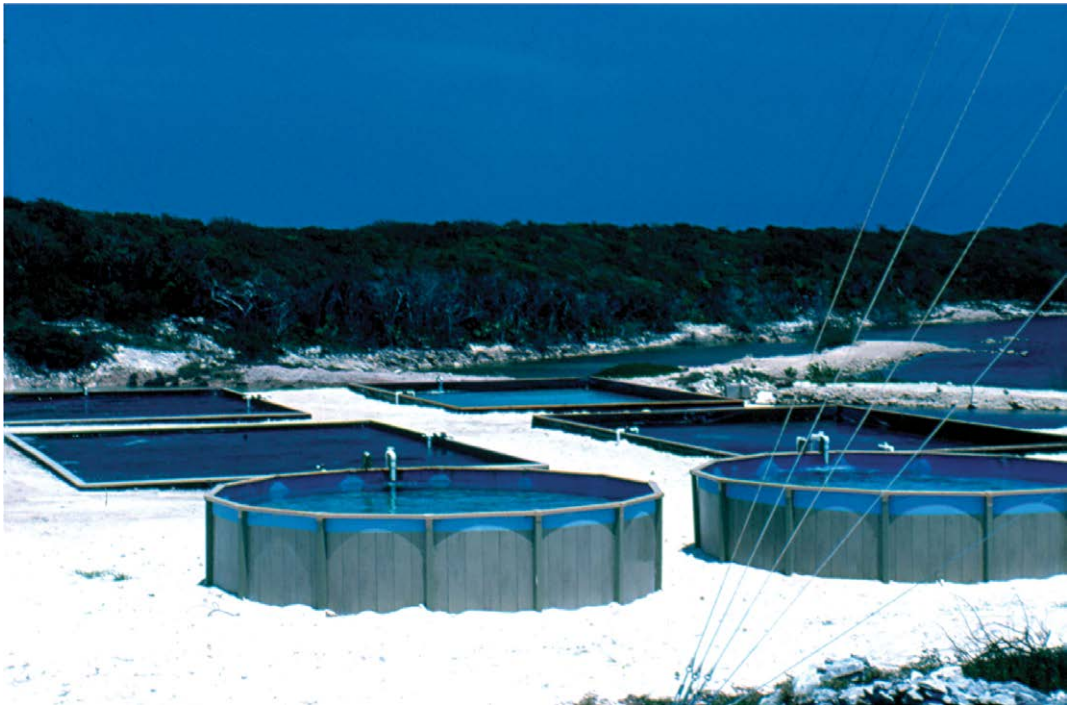
Fig. 3.14. Large circular tilapia growout tanks using seawater in the Bahamas.
