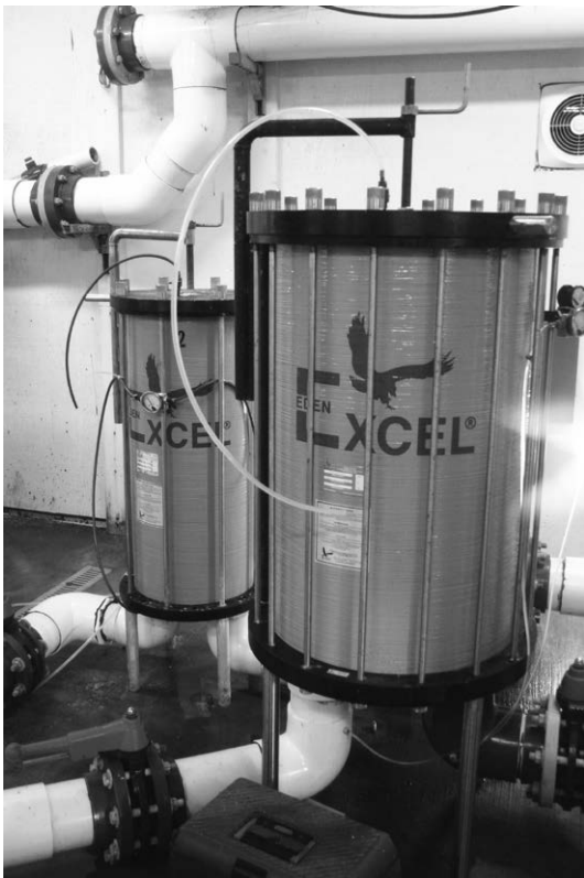
Fig. 3.24. A cartridge filter.
