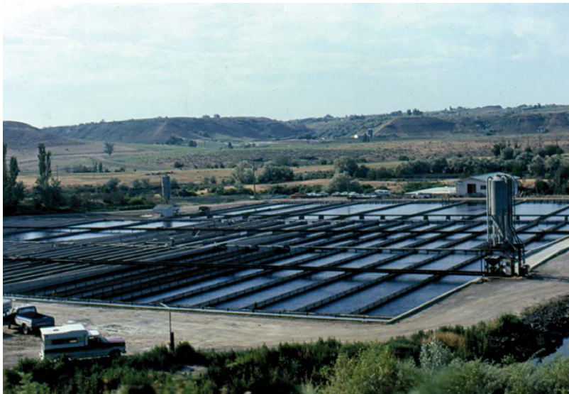
Fig. 3.12. Raceways at a commercial trout farm.
