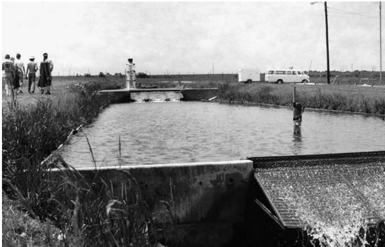
Fig. 3.16. Baffleboards between raceways provide aeration.
