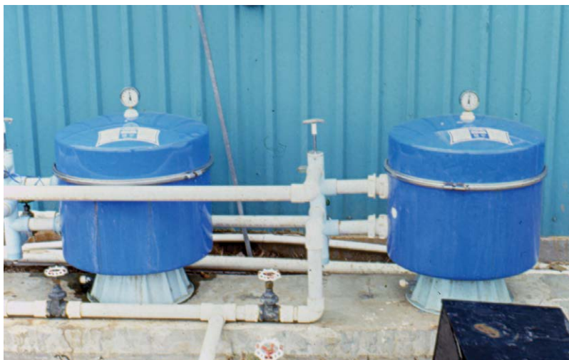
Fig. 3.22. A pair of sand filters.
