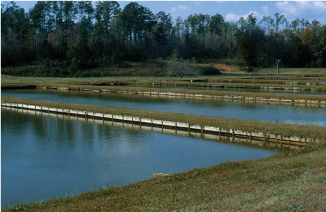
Fig. 3.1. An example of ponds with vertical reinforced side walls.
