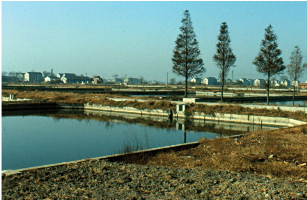
Fig. 1.5. Vertical walls and associated fencing in these ponds in the Philippines help keep walking catfish from escaping.
