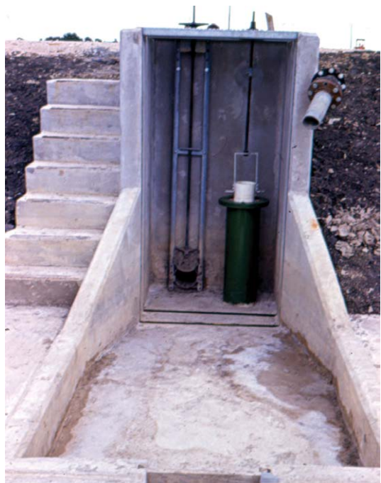
Fig. 3.10. A kettle drain structure.
