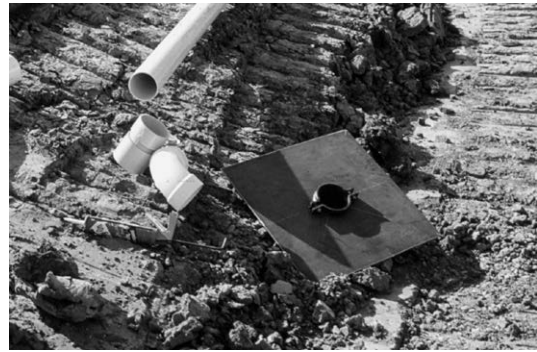
Fig. 3.8. A metal antiseep collar and some of the PVC components prior to being assembled.
