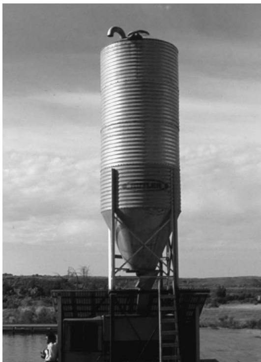
Fig. 8.12. Bulk storage bin for feed at an aquaculture facility.
